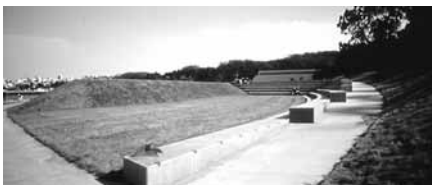
Figure 4. The West Bluff picnic area at Crissy Field was built with earth excavated to restore wetlands. (Photograph by M. Boland)
